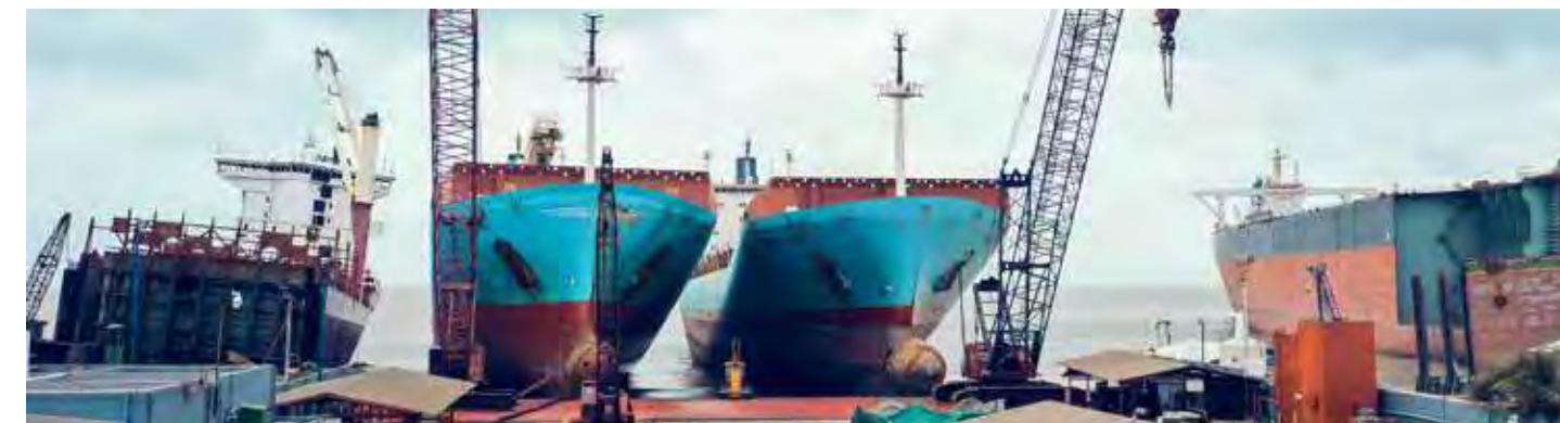
The Tove Maersk and MCC Halong undergoing responsible ship recycling at Y.S. Investments (Plot 59) in Alang, India – Sep '20.
